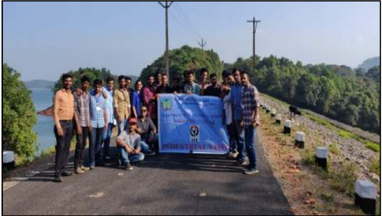
Fig. 49: Industrial visit to Varahi hydropower plant, Hosangadi and Mani dam, Yadur for final year students, on 25 February 2019, by the Industry Interaction Cell of Mechanical Engineering
