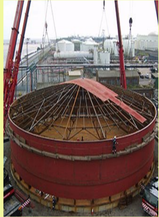
Figure 3: Fixed cone roof tank drawing with parts (Left) and Construction of Fixed roof tank (Right)
